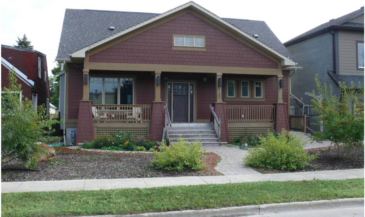
Figure 17: LEED Silver Rated Home, Winnipeg. This house was designed to be sustainable and highly energy efficient. Some green elements of the house are the use of reclaimed wood, a grey water recycling system, energy efficient fixtures and appliances, increased amounts of insulation and a low maintenance yard with drought resistant native plants.
