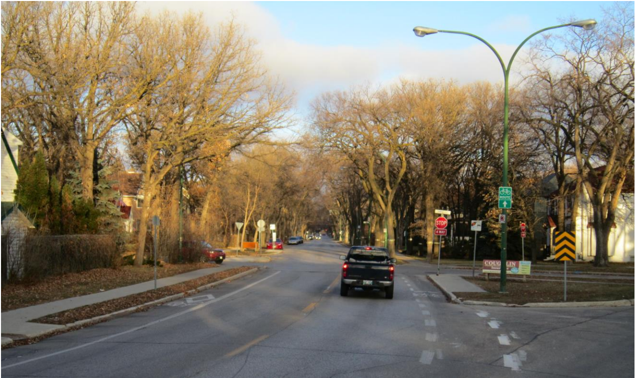
Figure 14: Bi-directional bike lanes, Winnipeg. Adding bike lanes to collector roads acts as the backbone for a strong cycling network and accommodates cyclists who are not willing or able to ride in traffic.
